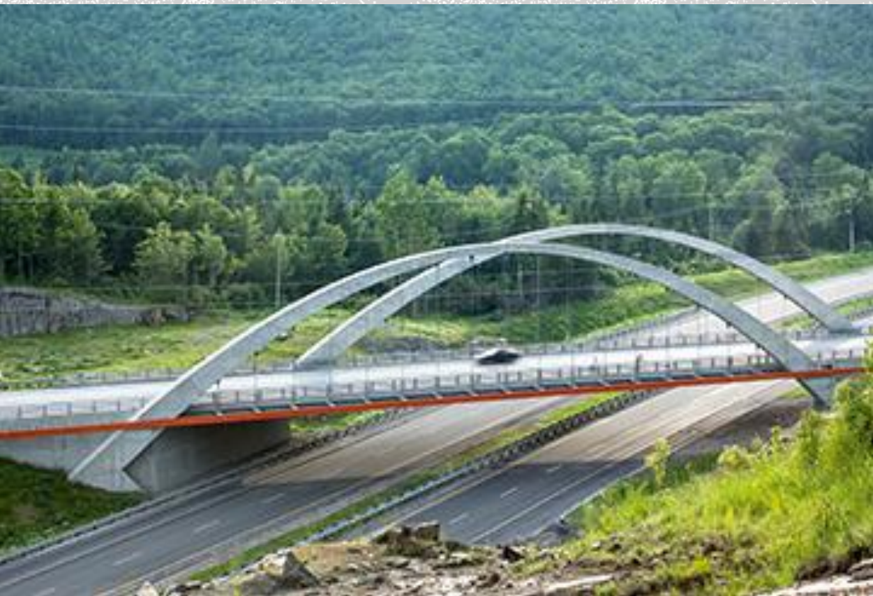
STONEHAM ARCH BRIDGE 2012, QUEBEC, CANADA
